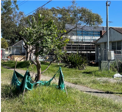
Street tree “protection”; it is worse up close! (Ph: P. Shelton)
