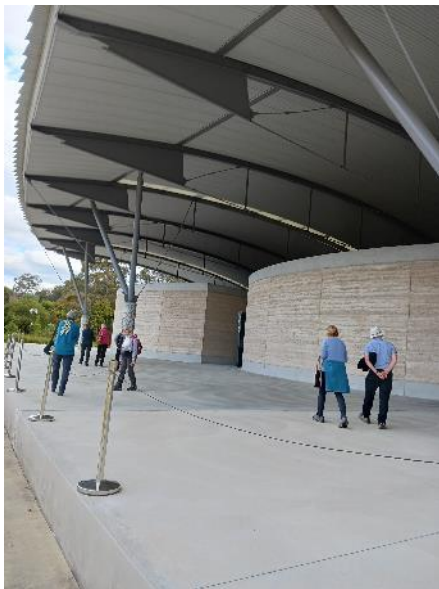
Members under fly-roof, along rammed earth walls of the Herbarium
