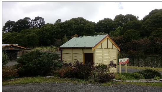
The 'lamp' shed today, looking across the railway line
