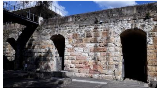
A massive sandstone platform with tunnels underneath
