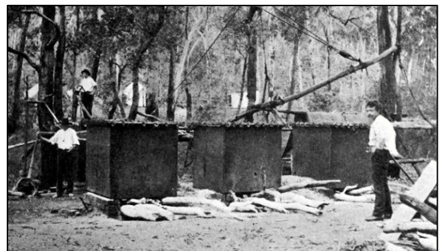
Direct firing, 3 tank Eucalyptus oil distillery plant at Wingello c.1910
