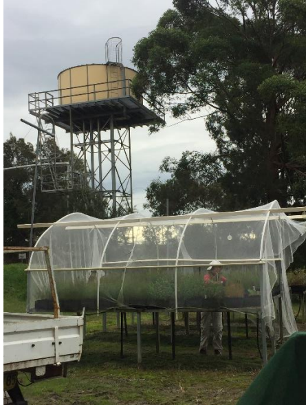
The overflowing tank, P Nagle.
