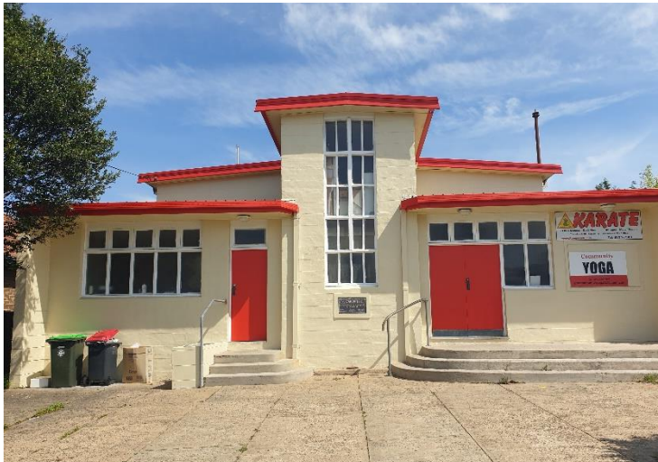
1 The Earlwood Uniting Church Hall
